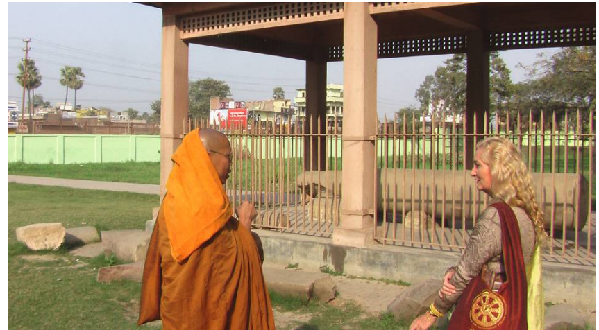
Badly shattered Ashoka Pillar – Patna
