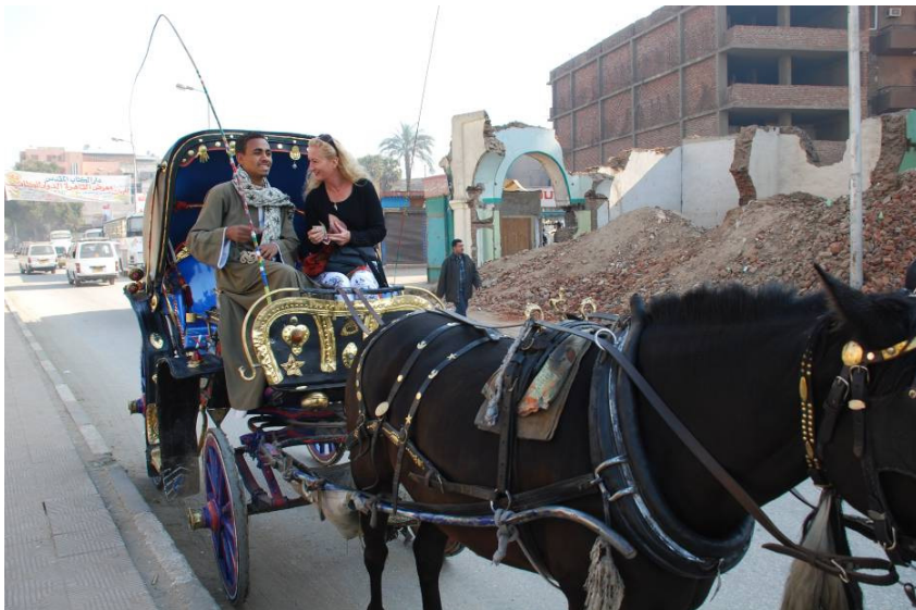
Calabash – Luxor Buildings being demolished to unearth more of the Avenue of Sphinxes Page 132
