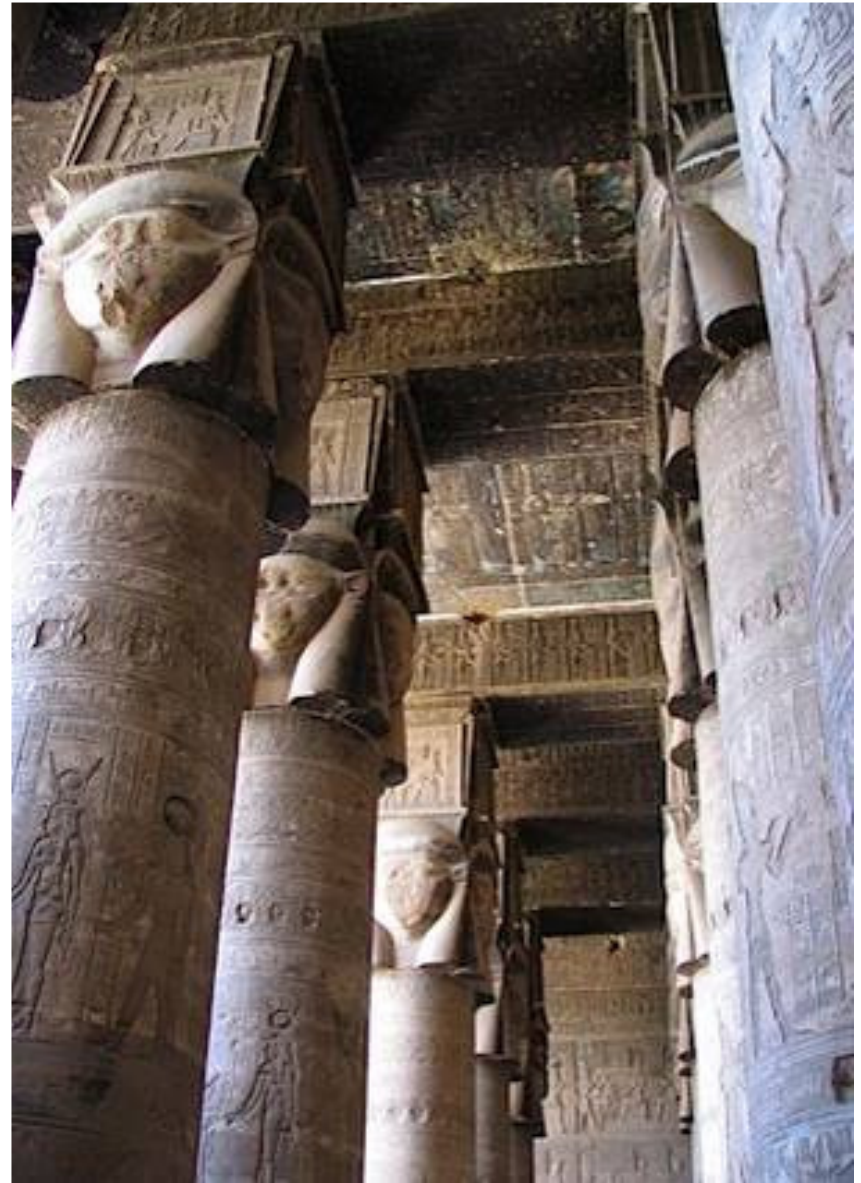
Damaged faces on the Hathor Pillars – Temple of Hathor – Dendera
